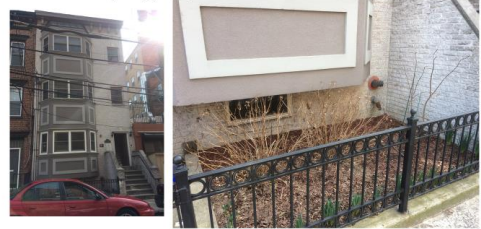
1. Landscaping adjacent to foundation
