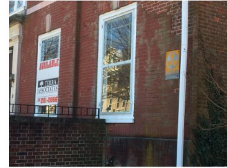
2. Basement window infill
