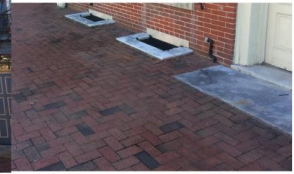
Exposed basement windows
