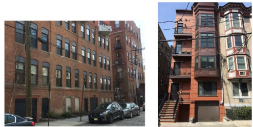
3. 1st floor abandoned; DFE residential use
