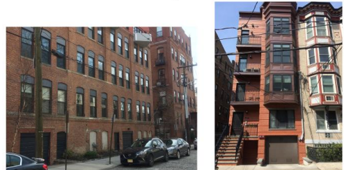
3. 1st floor abandoned; DFE residential use
