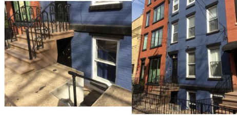
2. Basement window infill
