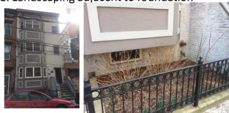
1. Landscaping adjacent to foundation
