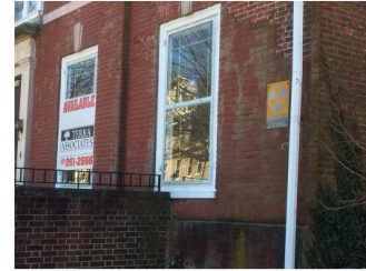
2. Basement window infill
